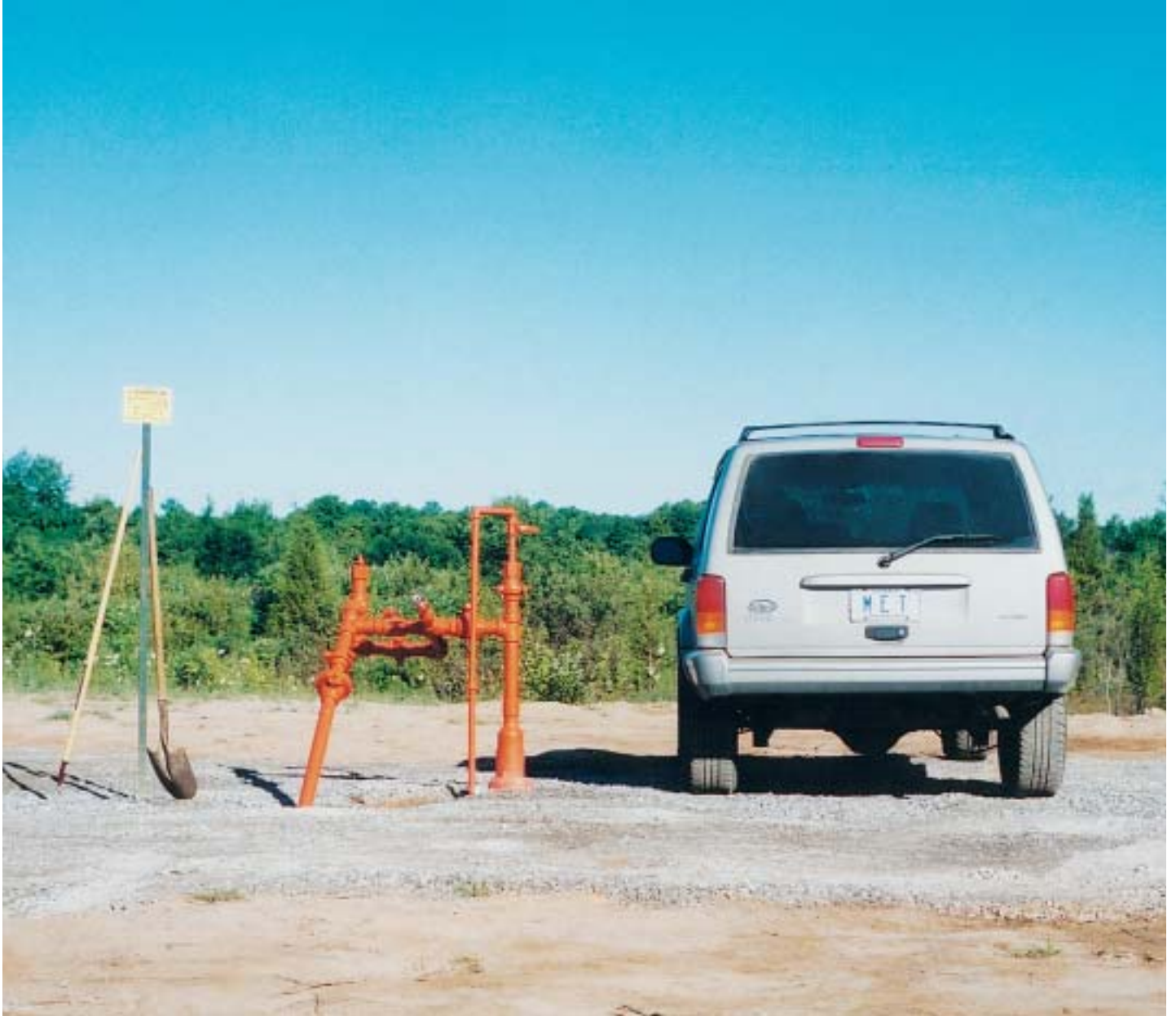
Producing Metalore SONG #8, Clear Creek Field, Houghton Township, Ontario, July/02.
